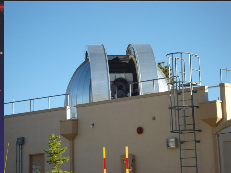
JPL's OCTL Facility in Southern CA
